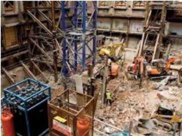
The project in Bartholomew Lane contracted **ASME** to install Rakers and Walers to support two floors of underground basement, whilst demolition work took place elsewhere in the building.
