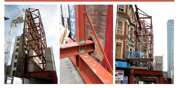
**ASME** supplied and installed internal and external facade retentions with tie systems to buildings 36, 40-42 and 48 Oxford Street. The works had to be completed over Christmas and at night using a crane for public safety due to high pedestrian traffic during the day.
